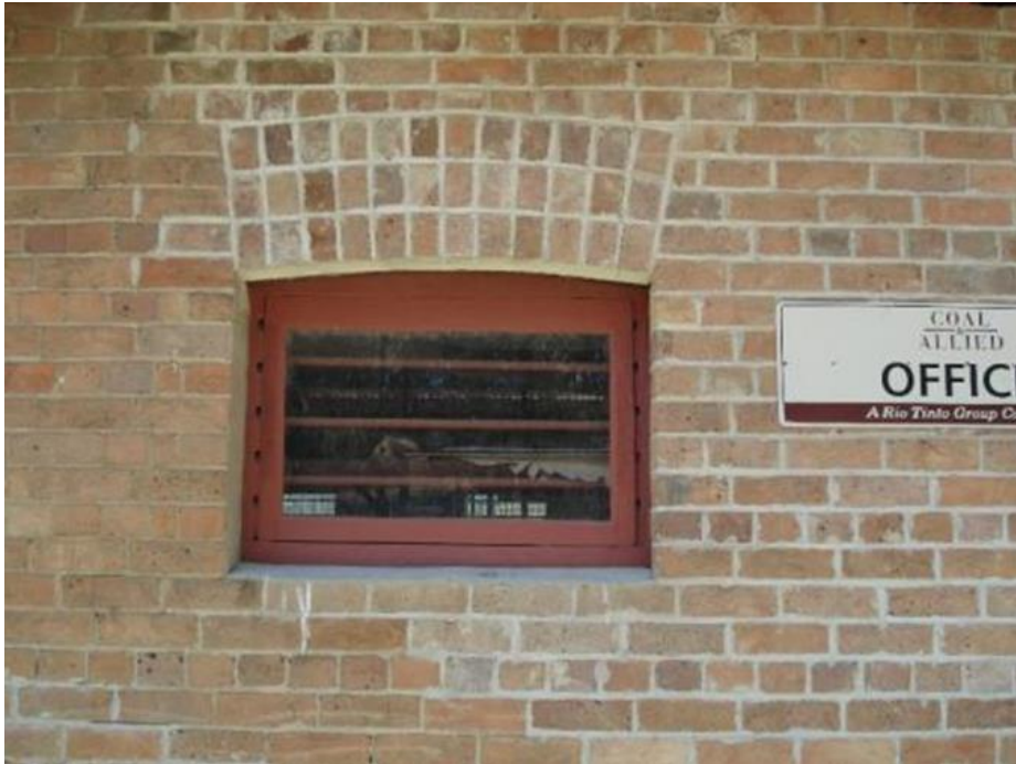
Plate 14 Window with row lock arch of three courses (RPS 2017)
