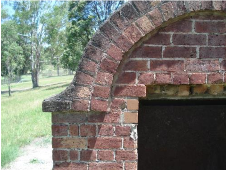
Plate 17 Detail of pitched brick vault (RPS 2017)
